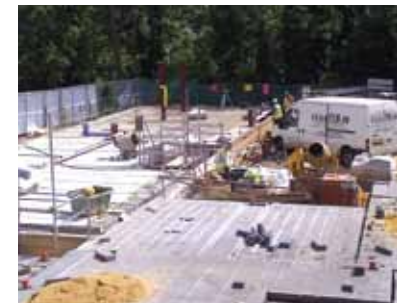
The building work for the new Haven in Holly Park, Islington
